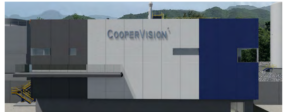
Above: A rendering of CVI Puerto Rico’s Combined Heat and Power plant
